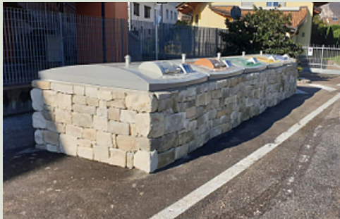
Semi-underground waste disposal centres. In 2023, ASIA - Azienda speciale per l'igiene ambientale, proposed the construction of partly underground waste disposal centres preventing access to animals as a solution to the problem of raids by large carnivores. These consist of containers in which waste is deposited at a depth of 1.5 metres below ground, also reducing odour emissions (the photo shows a waste disposal centre constructed at Mezzolombardo).
