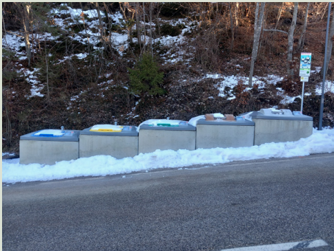
New semi-underground waste disposal centre at loc. Santel, Fai della Paganella. Work was carried out as priority A, in December 2024 by ASIA - Azienda Speciale per l'igiene ambientale. Waste disposal centre made up of 5 containers (organic, paper, packaging, glass and non-recyclable), of which three with a capacity of 5m 3 (non-recyclable, paper and packaging) and two 3 m 3 (organic and glass). The waste disposal centre shown is one of the 10 already built on the Paganella tableland. In spring 2025 they will be clad with natural stone.
