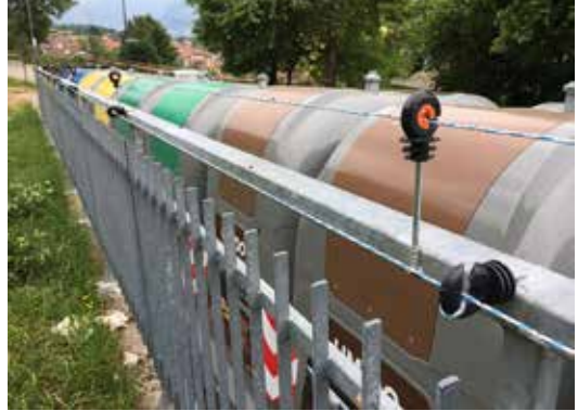
Photo 20 - Fai della Paganella: the same waste disposal site shown in the previous photos, equipped with a physical barrier on three sides and electrified wires (M. Zeni - APT Wildlife Department archives)
