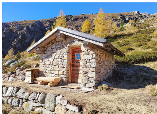
Photo 15 - Traditional stone shelter renovated in 2025 by staff of APT's Forestry Department at Laghi della Bella Venezia, Bieno. (R. Dalledonne, APT Wildlife Department archives)
