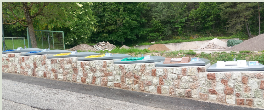
Photo 2 - Waste disposal centre made up of 7 semi-underground containers in the Municipality of Fai della Paganella; work carried out by A.S.I.A. srl.
